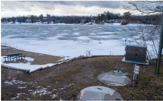
Five lift stations that service Lake in the Hills Sanitary District. Systems are custom built to meet the specifications of each site. Each system arrives at the site pre-wired, pre-tested, and ready to go.
