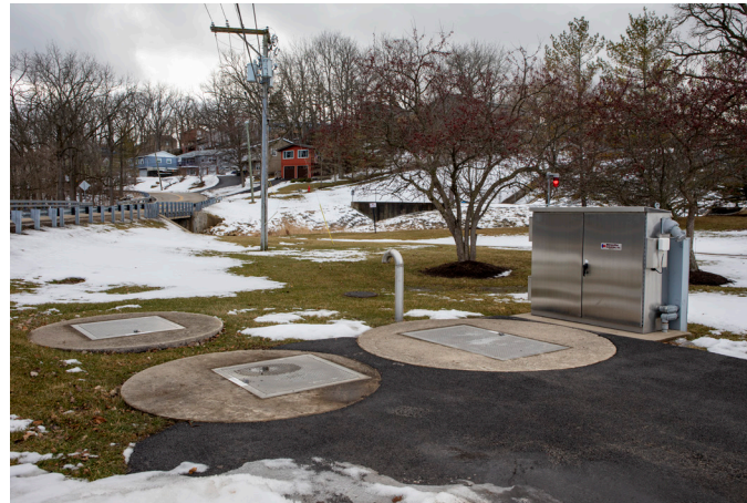
Five lift stations that service Lake in the Hills Sanitary District. Systems are custom built to meet the specifications of each site. Each system arrives at the site pre-wired, pre-tested, and ready to go.
